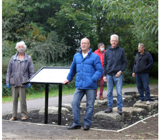
BIG finishing their new installation opposite the Masons Arms in Shildon on the route of the S&DR
