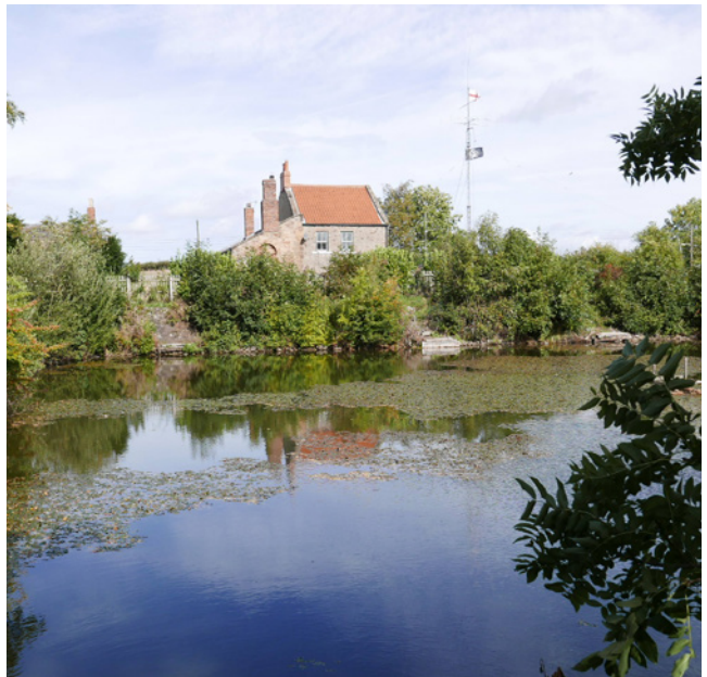
Brusselton Engine House and Reservoir
